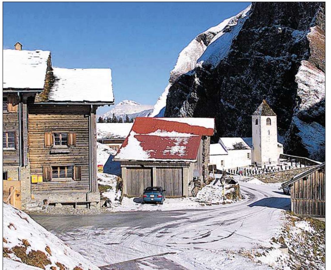
Thalkirch. La part dadens da la Val Stussavgia cumpiglia plirs aclaus e bains isolads.
